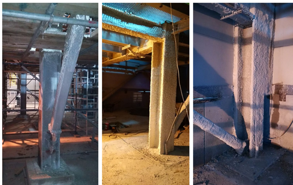
Figure 2. Steel structures with the fireproofing plaster compositions.
